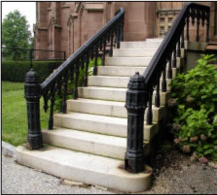
The Cathedral's exterior remains in excellent condition, considering the porous nature of its Belleville brownstone. Some weathering has taken place, as seen in this stairway.
