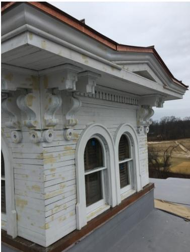
5. After refurbishing and reconstructing the elements of the cupola, and installing the new materials, Old World Quality workmen readied the cupola for priming.
