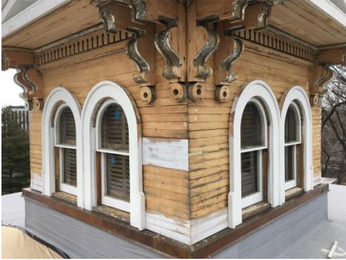
3. Window trim and sashes restored with new materials to mirror the original architecture were installed.
