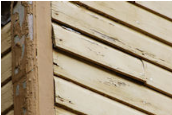
Above: Delaminating clapboards and exposed corner boards Near right: Wall junction showing rotted and separated siding trim Far right: Rotted ballister
