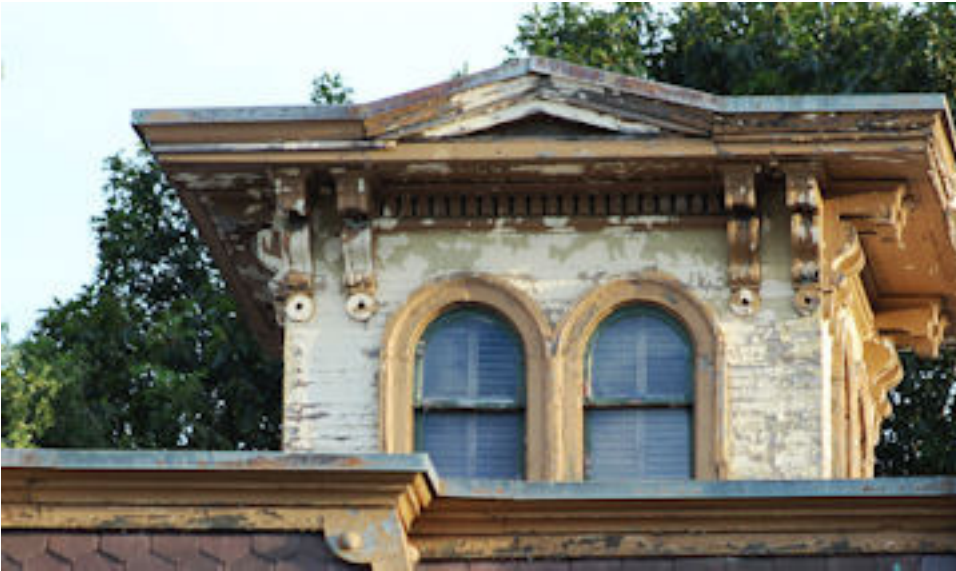
Left: Weather beaten and deteriorated window sashes, soffits and brackets on Widow's Walk Above: Peeling decorative trim
