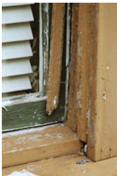
Above: Delaminating clapboards and exposed corner boards Near right: Wall junction showing rotted and separated siding trim Far right: Rotted ballister
