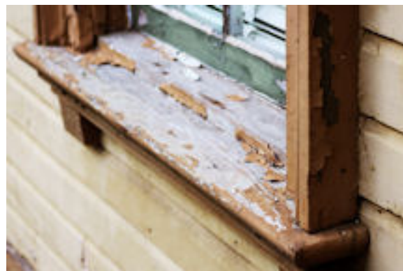
Windows and sills: Typical weather damaged and exposed windowsill and trim; separated boards and braces
